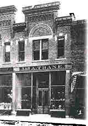
Trane Storefront La Crosse, Wisconsin 1891
